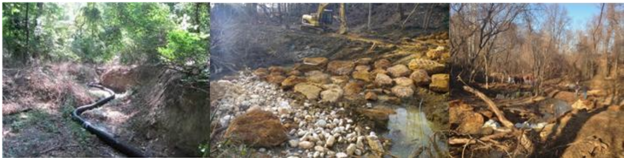
Figure 4. Pictures of the process of implementing RSCs in the headwater channels and in the main channel of Cabin Branch. The plastic tube used to diverge streamflow is shown on the left. The middle picture shows rocks and boulders used to build weirs across the channel. Tree trunks and other wood debris (right picture) are also used modify the stream discharge.
