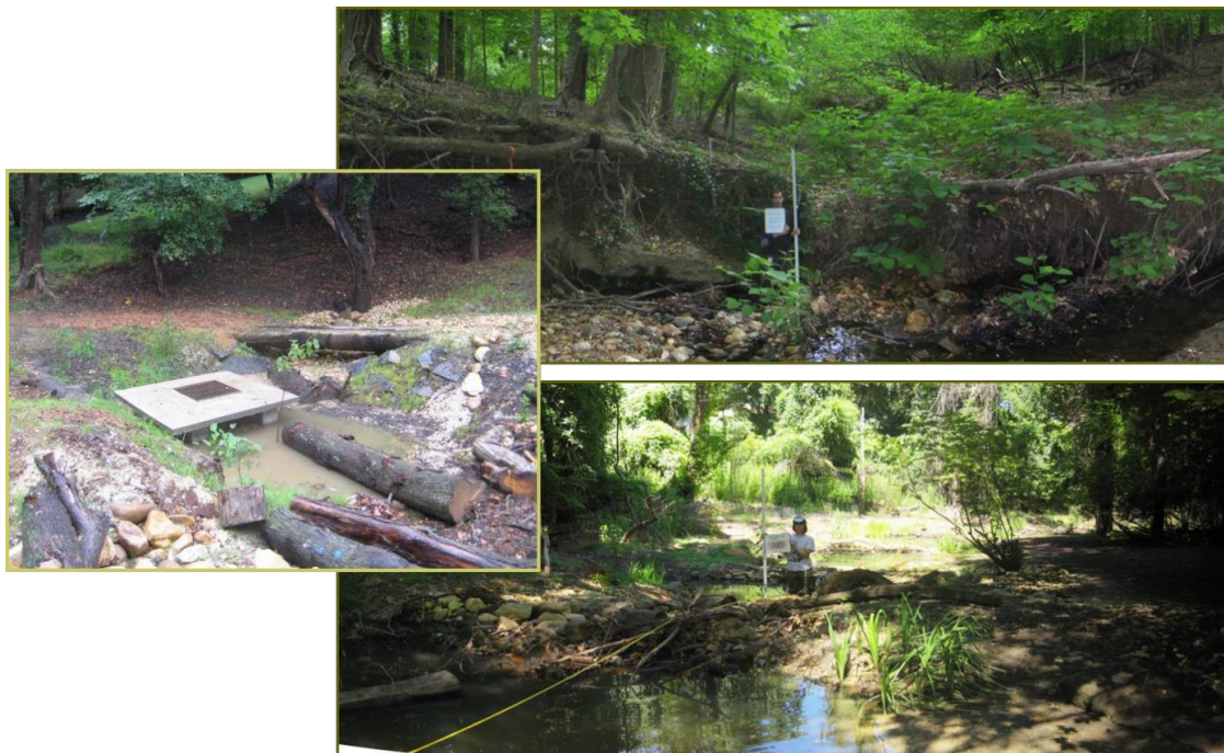
Figure 9. Pictures of before (top) and after (bottom) restoration implementation. The bubbler system is shown on the left. The stream previously began at an outfall pipe which was buried as part of the project and retrofitted with a bubbler.
