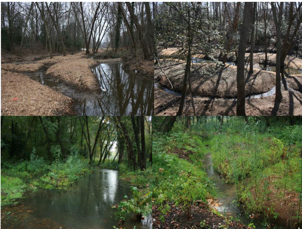
Figure 8. Meandering anastomosed channels separated by floodplain islands. The photos on the top were taken immediately after construction and the photos in the bottom were taken in the summer, one year after the end of construction.
