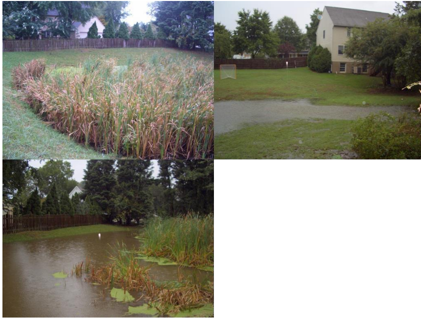
Figure 14. Picture of Dunkeld Manor stormwater structure before retrofit implementation (top and bottom left); picture of flooding problem in the adjacent residential area (top right).
