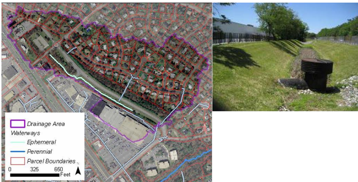
Figure 12. Aerial photo (left) with the delineation of the drainage area associated with the RSC implementation to substitute the old structure (grass swale above).
