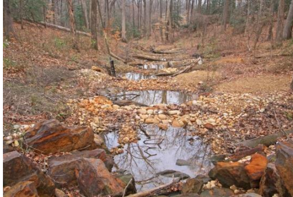
Figure 4. Step Pool Stormwater Conveyance system with its series of step pools separated by berms along a downhill slope.
