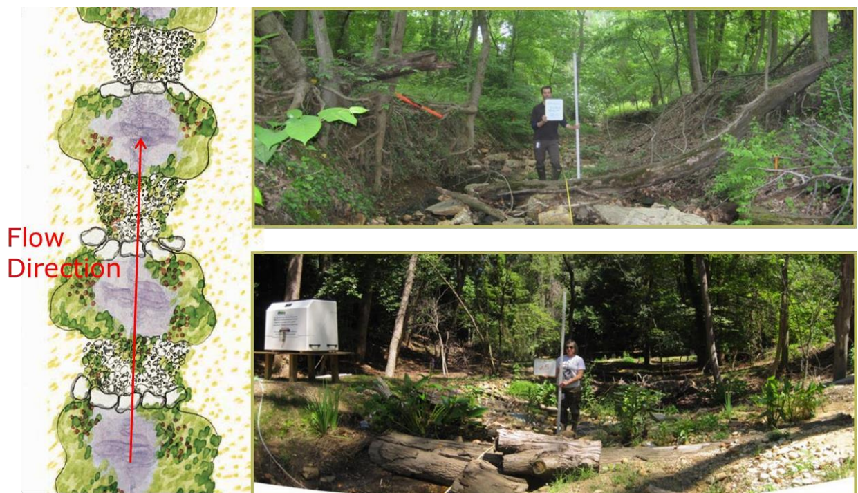
Figure 8. Schematic of an RSC (left) and pictures of before (top) and after (bottom) restoration implementation.
