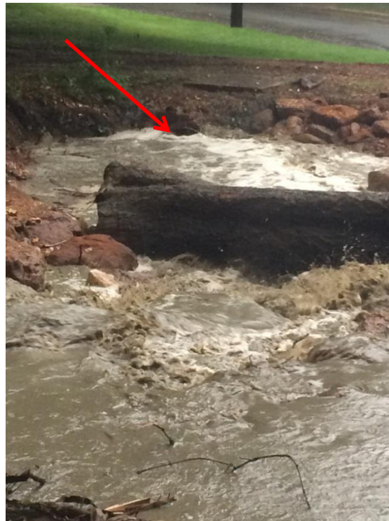
Figure 8. Photo of the 41" diameter RSC outflow (arrow) virtually submerged during a large storm event (1.7") on July 10 th , 2014. TSS concentrations in this runoff, which was during the construction period, exceeded 3.6 g/L
