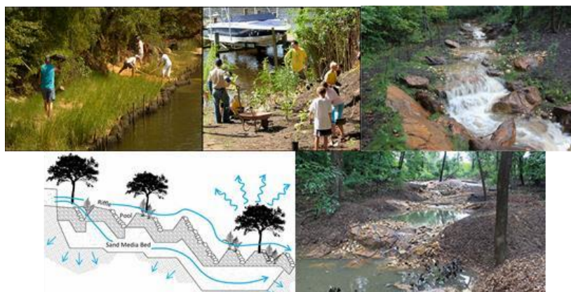
Figure 5. Types of projects designed to prevent erosion and the export of sediments into tidal waters. They include restoration of living shorelines (top left and middle), and Regenerative Stormwater Conveyance systems replacing conventional stormwater conveyance structures (top right and bottom pictures).
