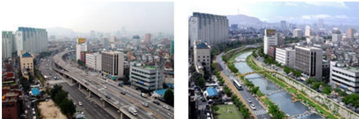
Figure 2. The highway built above the river that was demolished as the first step in the restoration project (left); an aerial view of the restored river.
