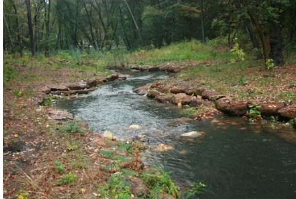
Figure 7. Picture showing a modified channel reach armored with rocks to enhance bank stability and provide sinuosity.
