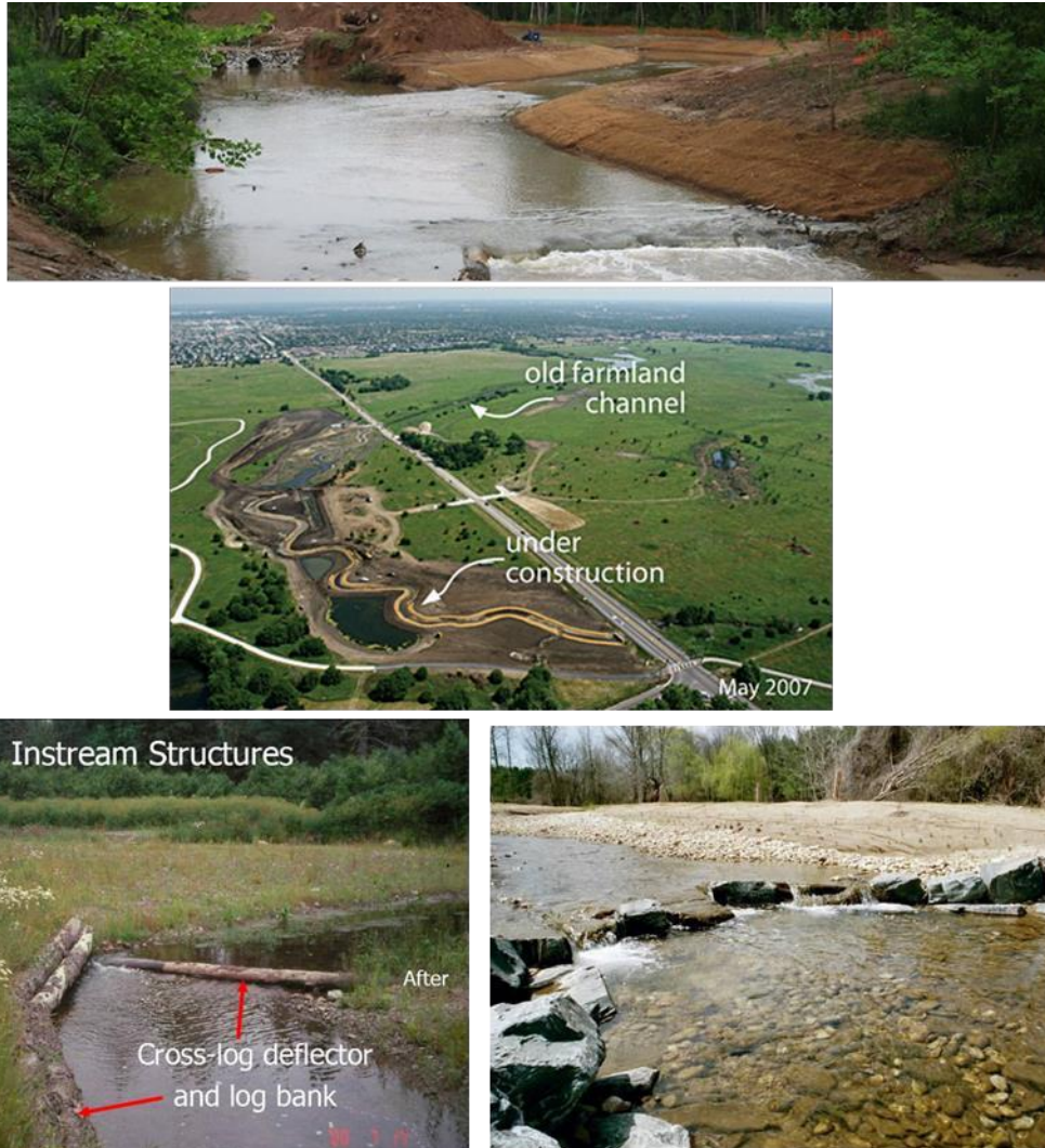
Figure 3. The most commonly used restoration practices are changes in the river channel (top two) or changes inside the channel (bottom).
