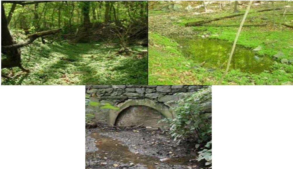
Figure 6. Portion of Broad Branch piped underground (top pictures). The pipe had been closed with a wall, which will be removed as part of the daylighting project.
